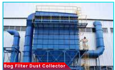
Bag Filter Dust Collector
