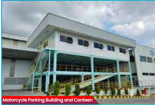
Motorcycle Parking Building and Canteen
